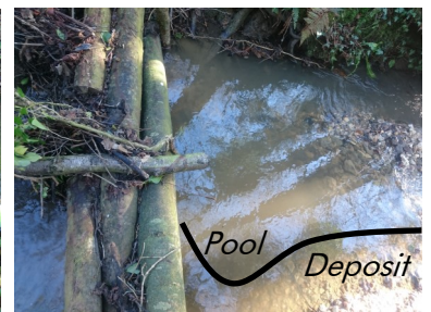
Left: October 2017, Right: Created scour pool and deposition of coarse sediment downstream February 2018.
