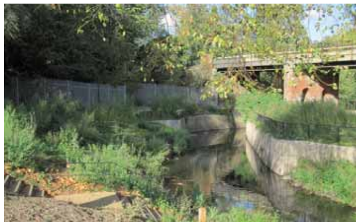
Regrading at waters edge and timber deflectors fixed to the concrete bed
