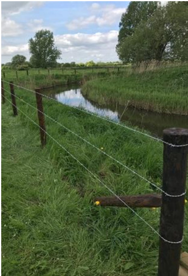
Figure 4 New fencing installed at Elton
