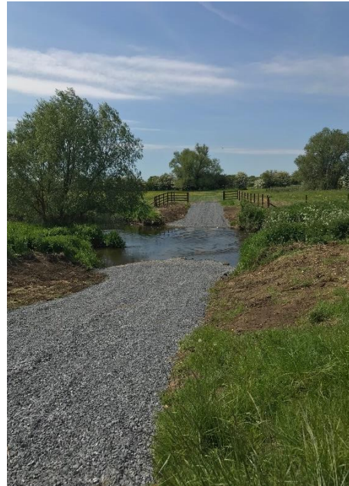
Figure 3 Elton ford after the works had been completed
