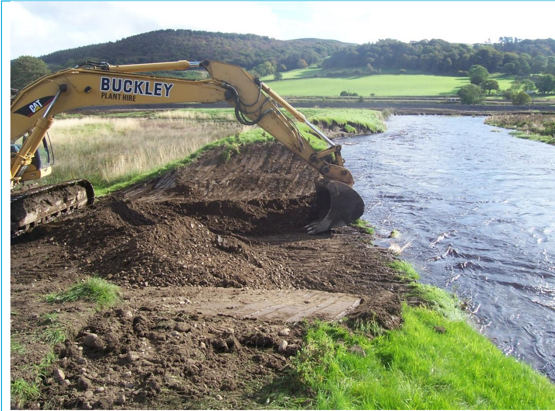
b) Inlet to paleo feature during construction showing exposed gravels at the bed level.
