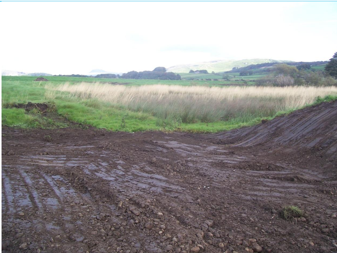
c) View from inlet into the paleo feature showing that the level of the inlet is set at approximately the same bed level as the paleo feature.
