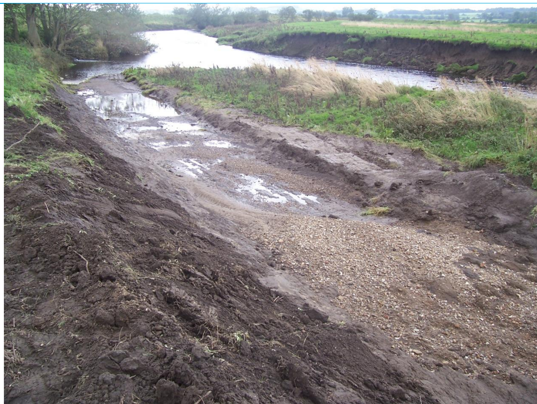
b) Downstream end of chute channel showing gravels exposed during excavation.
