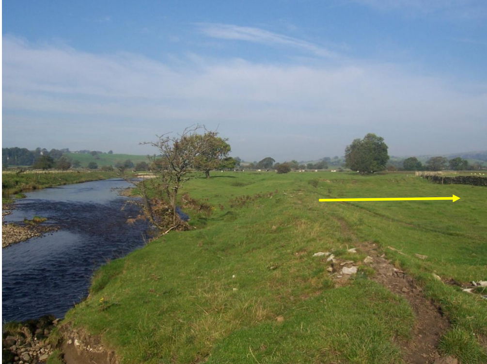
Figure 3-3: Flood embankment that could be set back over left bank
