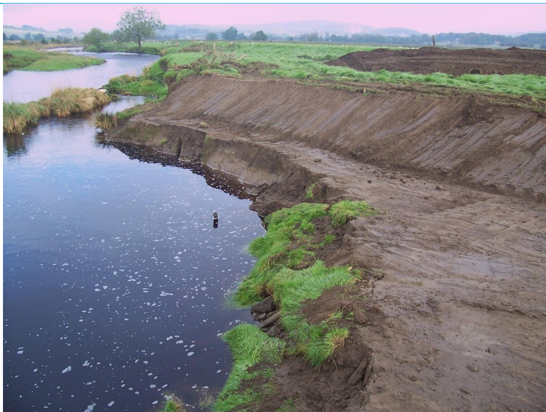
b) Upstream inlet to chute channel (note - entrance angle has now been smoothed off
