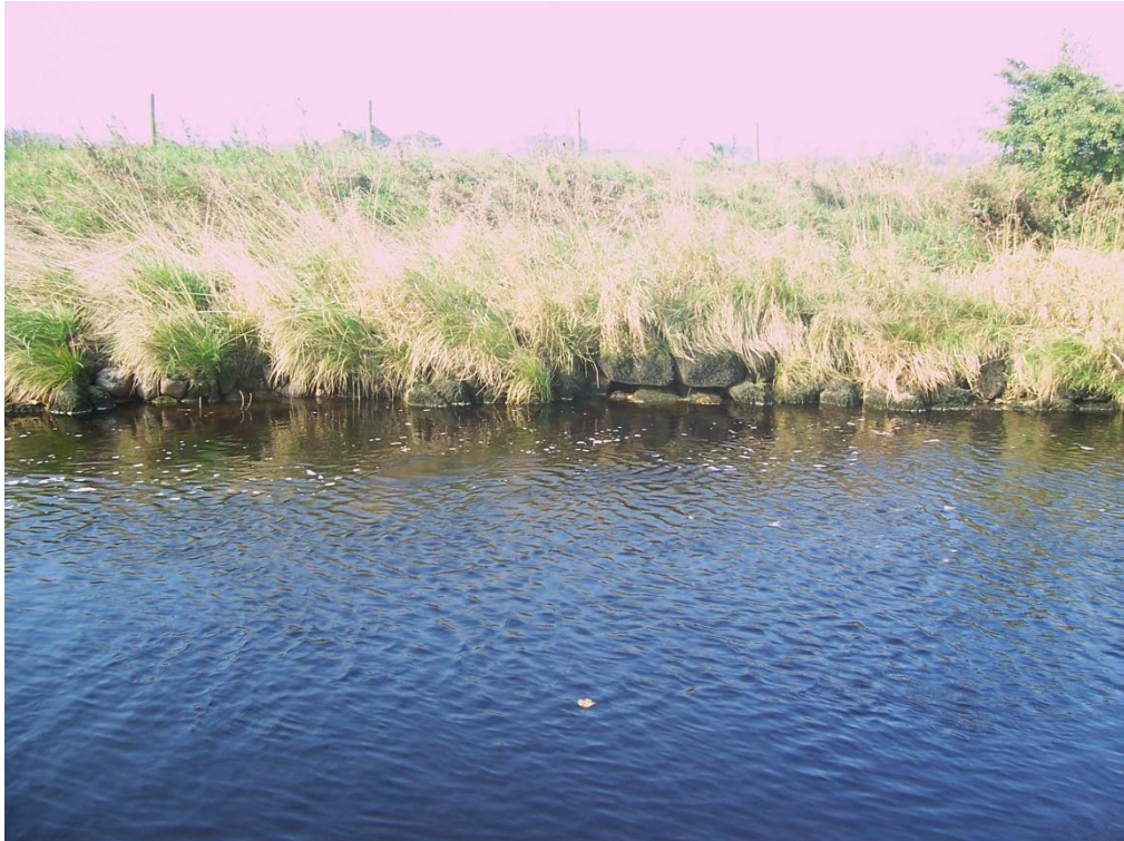
Figure 3-4: Potential revetment removal on right bank
