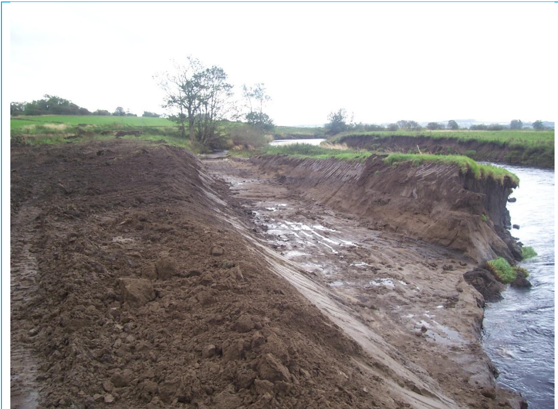
a) View of chute channel looking downstream. Note the water level marks on the right bank of the chute channel showing level of recent flood.
