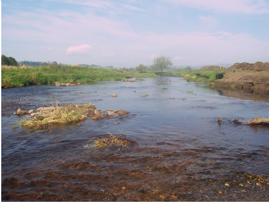
b) Boulder cluster network and bed coarsening looking downstream (note flow variation improving the diversity across the uniform glide).
