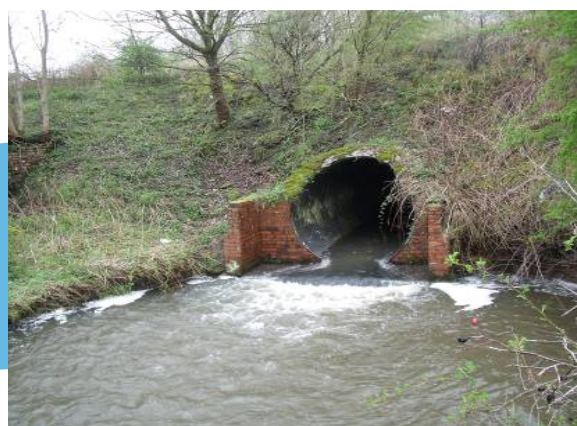
Figure 2 - Original erosion pool and concrete step
