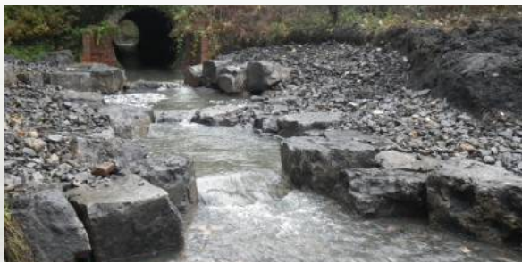
Figure 4 - Completed rock ramp easement
