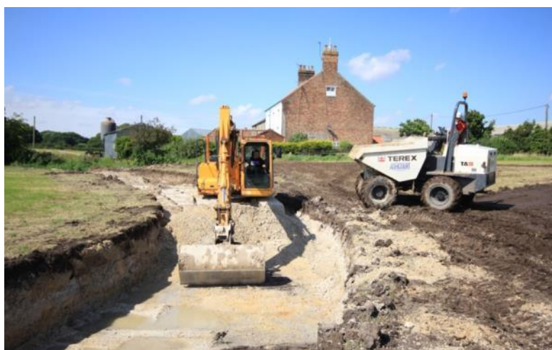
Channel forming with the chalk substrate visible © East Yorkshire Rivers Trust
