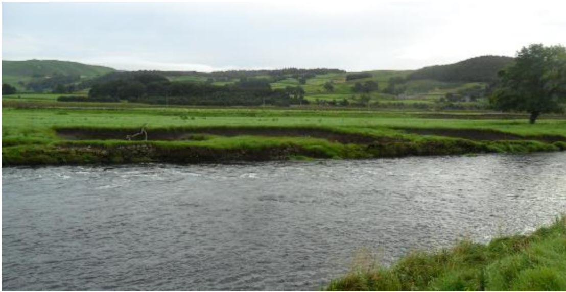
Figure 9. Retained revetment along the River Ribble.
