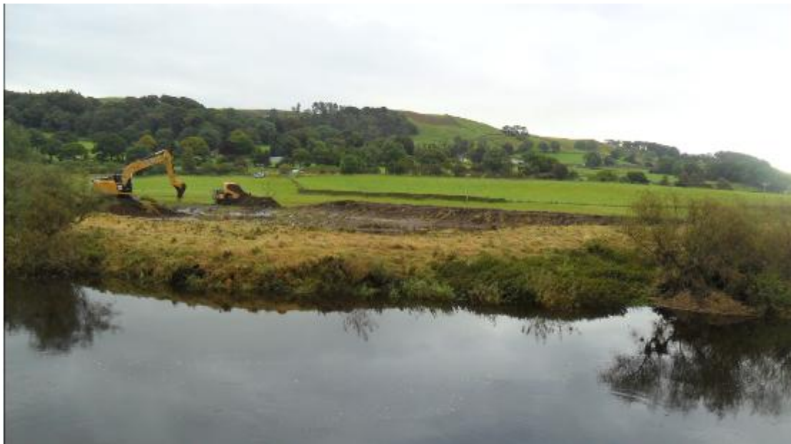
Figure 15. Construction of floodplain scrape on the River Ribble.
