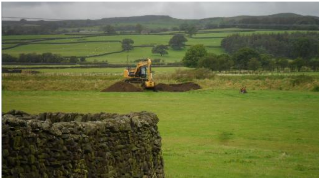
Figure 13. Flood bank realignment on the River Ribble.
