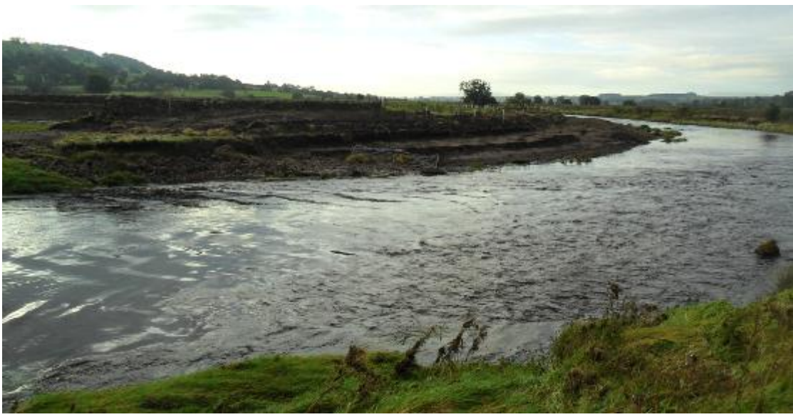
Figure 3. Lower left bank reprofiling on the River Ribble.
