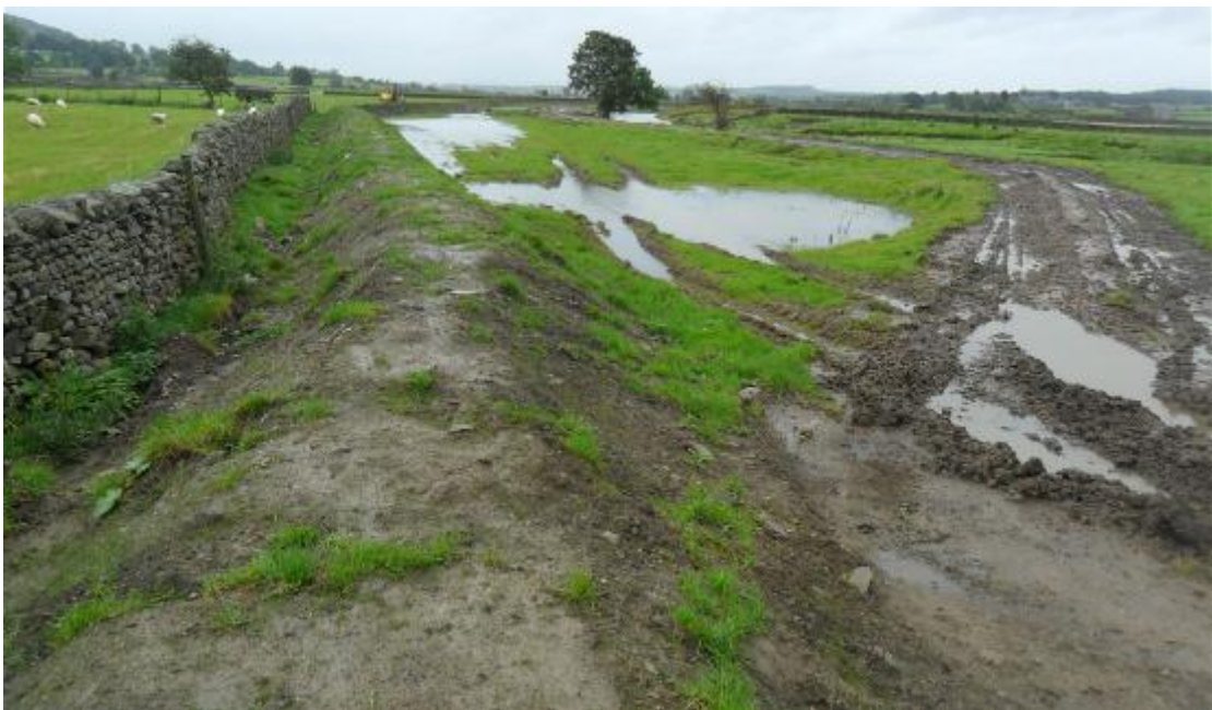
Figure 8. Left bank flood bank realignment showing reconnected floodplain.
