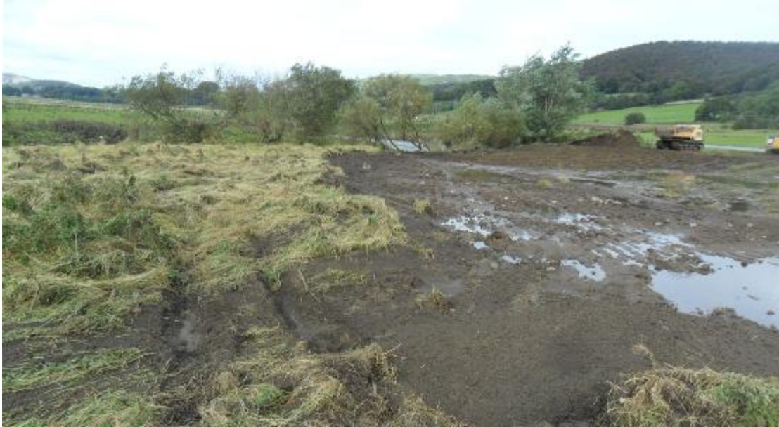
Figure 14. Construction of floodplain chute on the River Ribble.
