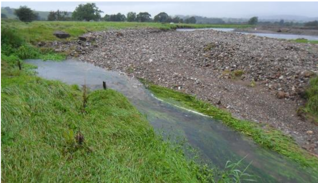
Figure 4. Chute channel creation on the River Ribble.
