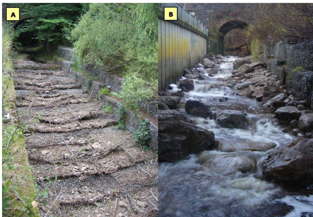
Figure 6: Replacement of gabion mattress with cobble pool-and-cascade, Inchewan Burn, Birnham. A: Before. B: After.
