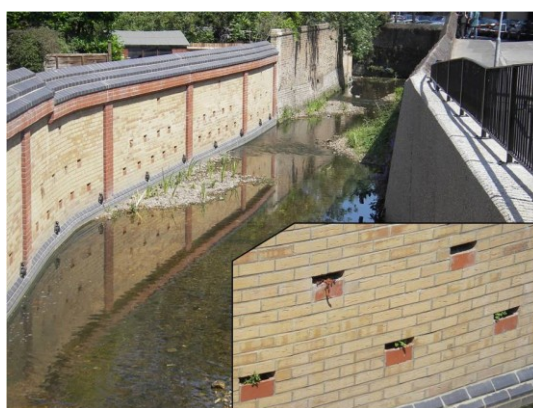
Figure 1: Flood defence wall with planting niches. River Quaggy, Lewisham
