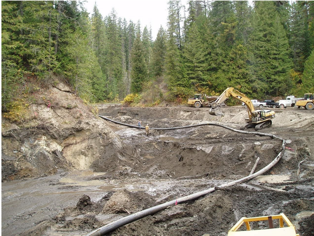
Figure 11: Sediment removal operation, with diversion pump line visible
