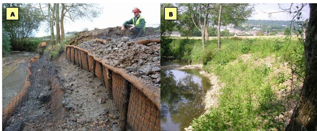
Figure 8: Back-filled coir net terrace revetment, River Char, Charmouth. A: As built, in 2005. B: With vegetation establishing, 2006.
