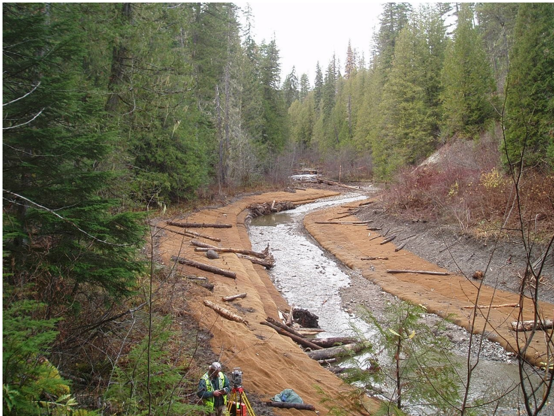
Figure 12: Coir matting bank protection (later planted out with native species), with coarse woody debris added to dissipate energy and increase flow diversity
