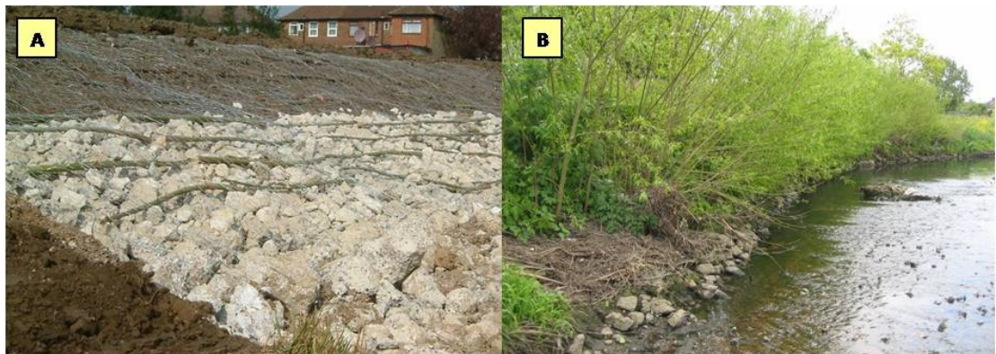
Figure 3: Crushed concrete and willow pole revetment A: as installed, in 2003; and B: with vegetation establishing, in 2005. River Brent, Willesden.
