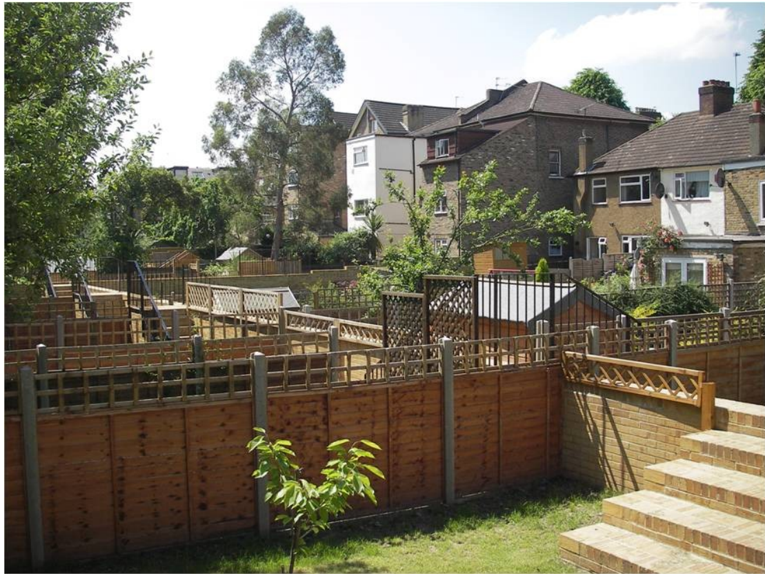
Figure 2: Flood defence wall set back and incorporated into gardens. River Quaggy, Lewisham.
