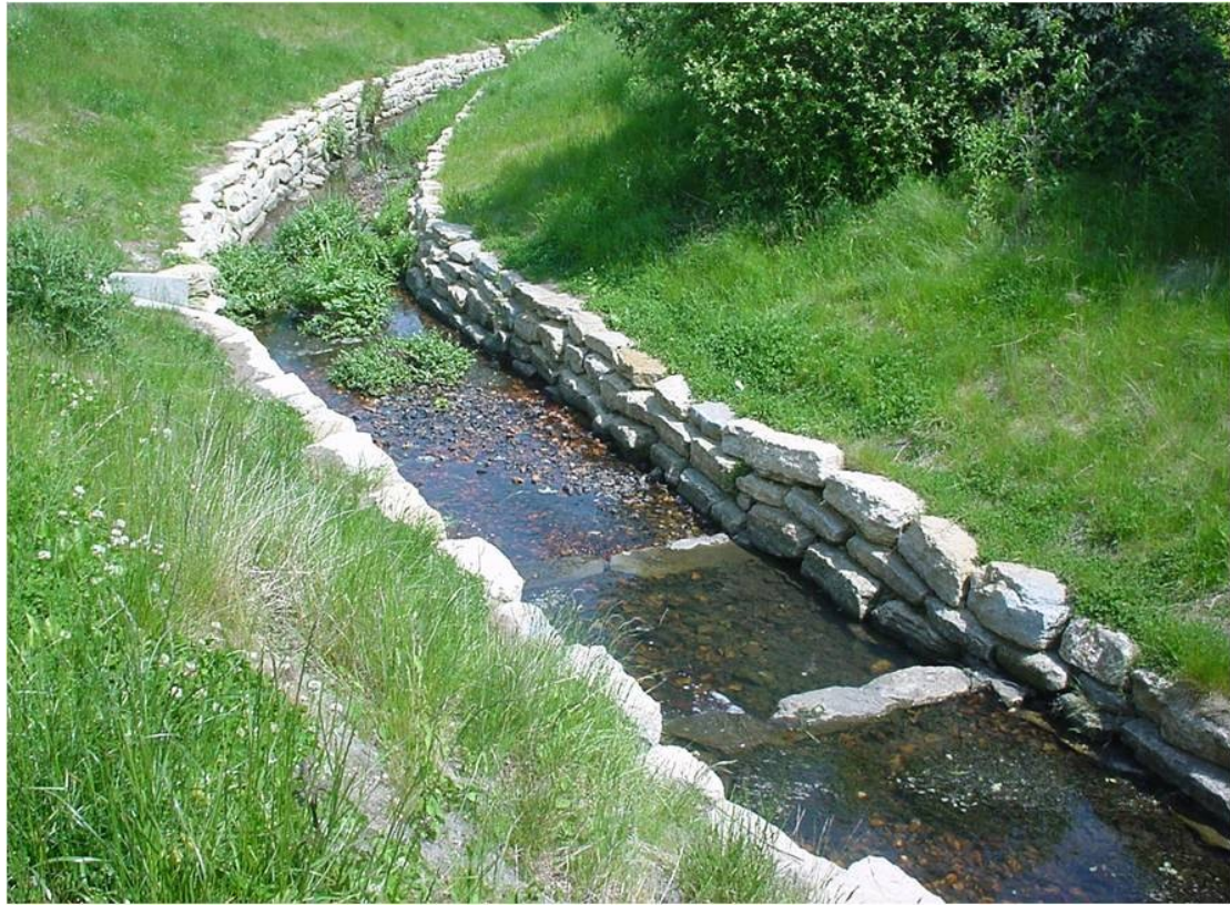
Figure 5: Small 'check weirs' on Tilmore Brook, Petersfield. Note the gravel being held behind the structures.
