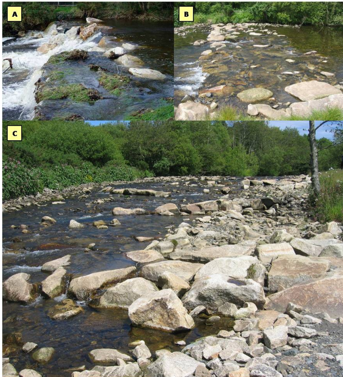
Figure 4: Rock ramp installed behind a dilapidated weir on the River Neb, Isle of Man. A: Weir before works. Photograph: Dept Transport, Isle of Man Govt. B: Partially drowned-out weir after installation of ramp. C: View of ramp, looking upstream.
