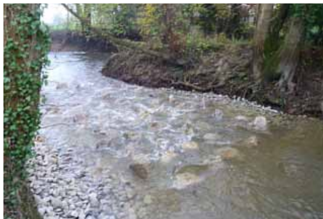
Rock ramp after completion of works
