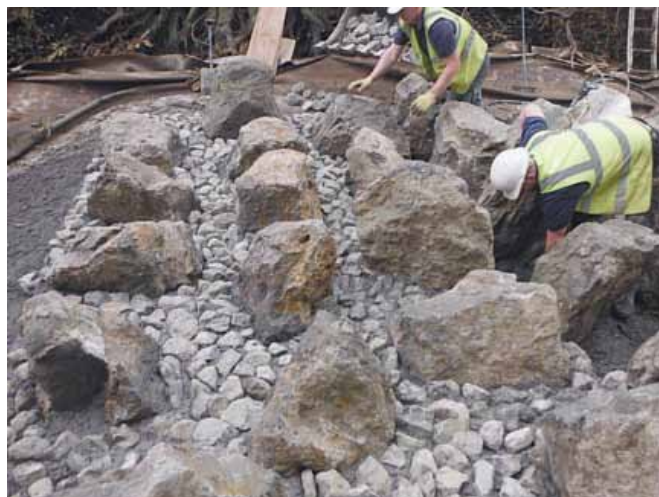
Rock ramp during construction
