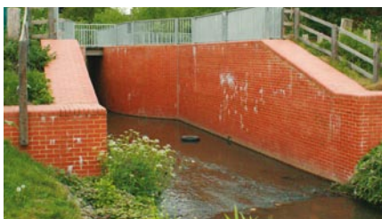
This flume was created in the river to divert floodwater into the sports fields at Weigall Road
