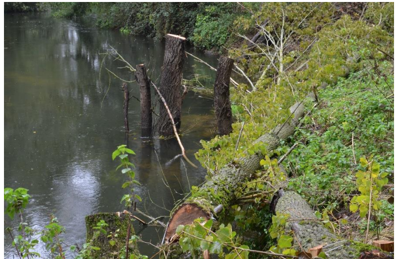
Figure 2 – Secured limbs on the bankface extending on to the channel
