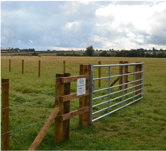
Figure 5 - Access gate on the new fence line
