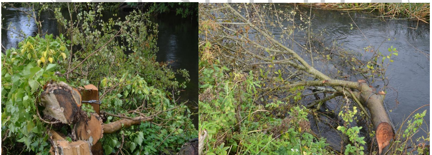
Figures 3 & 4 – Smaller hinged and pinned trees extending in to the channel
