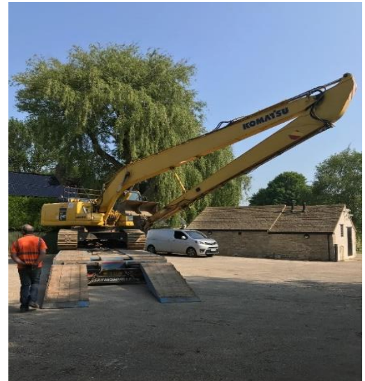
Figure 3 4– 20m long reach excavator for placing the gravel in the channel
