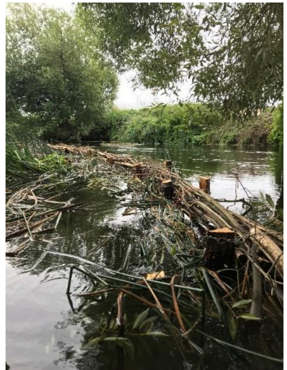
Figure 5 Faggot bundle revetment mid-channel to deflect flow
