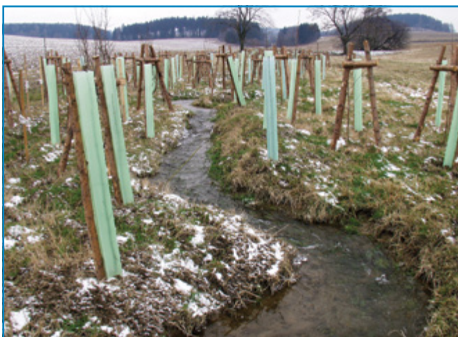
Fig. 2. Restoration (1999, 2000) of two formerly channelised streams in the middle of arable fields, Dolní Moravice, N Moravia. After removing the concrete tubes and filling the grooves, a shallow, varied streambed and several retention reservoirs were created with an excavator. Subsequently autochthonous trees were planted in the space between the reservoirs to create a local biocorridor. This operation was initiated, designed and realised by Ekoservis Jeseníky, Světlá hora and financed from Landscape management programmes. (L. Bureš)
