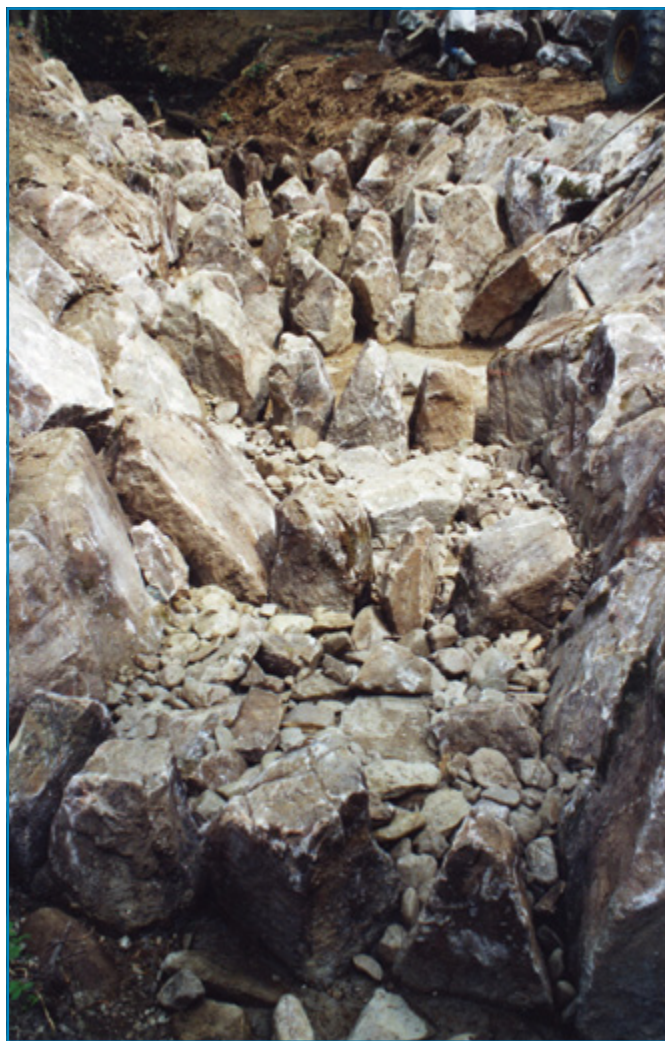
Fig. 5. Bypass under construction. Depositing of coarse gravel on the stream bottom between the stone sills. (V. Šámal)
