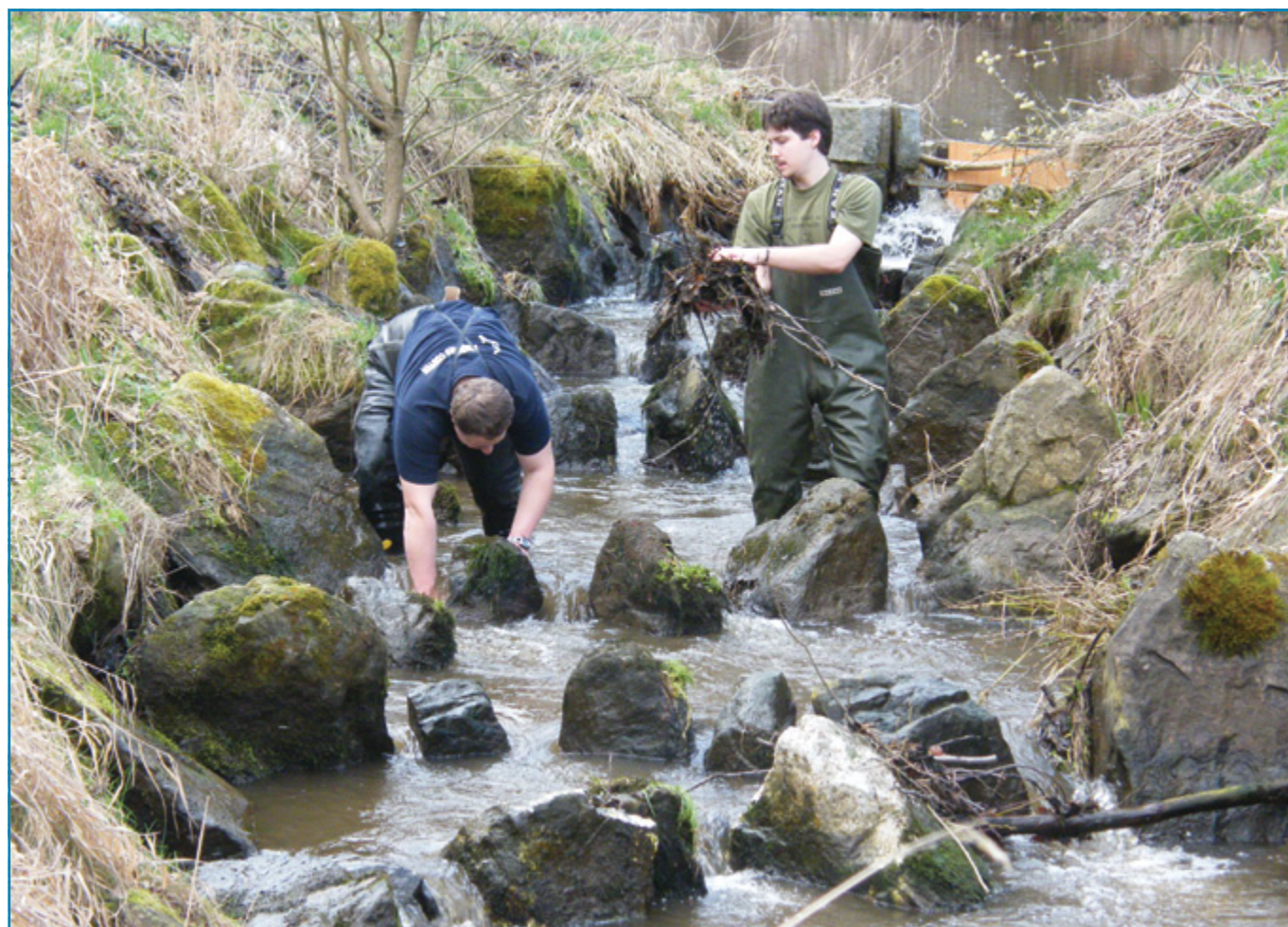
Fig. 4. The bypass under construction. Depositing of boulders on the banks and into the sill across the stream. (V. Šámal)
