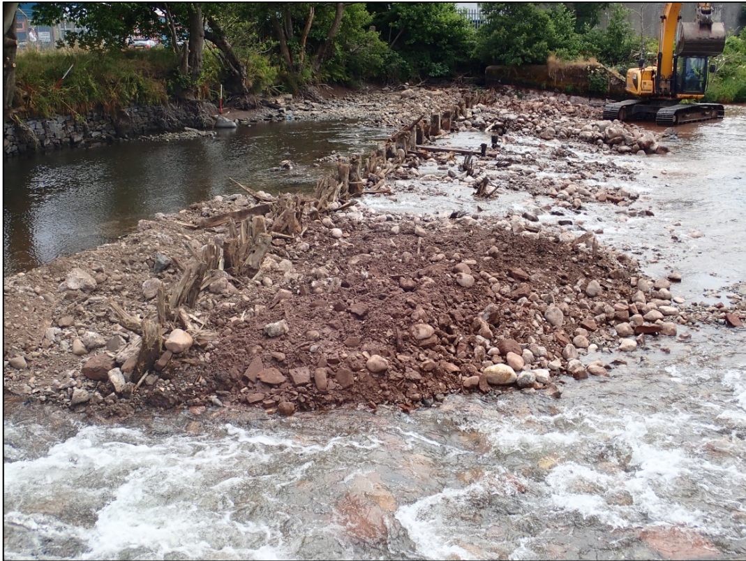
Photograph 13: Gravel and smaller cobbles forming the main body of the weir, looking south
