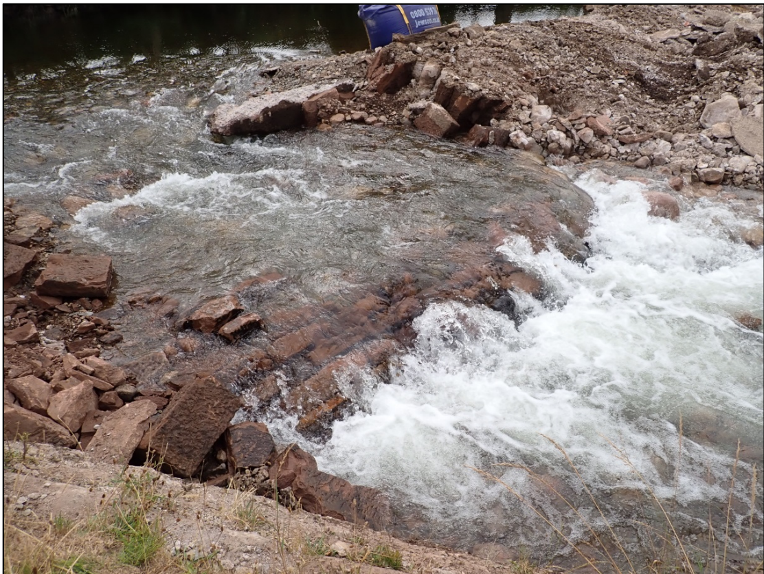
Photograph 2: Notch cut through the weir, with lower course of sandstone visible under water and upper course visible in section, looking south
