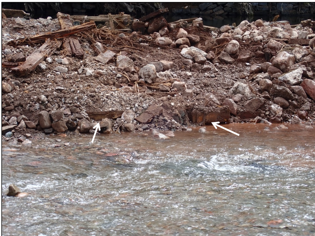
Photograph 12: Planks set on edge forming the rear (west side) of the weir, looking east
