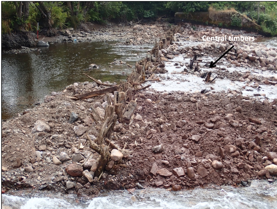
Photograph 11: Front upright posts and remains of central upright posts, looking south
