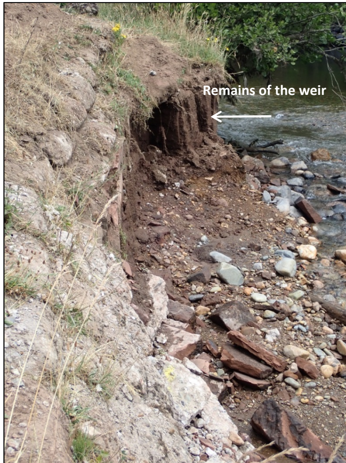
Photograph 9: The remains of the sandstone part of the weir, sat against the bank reinforcement, looking north-east
