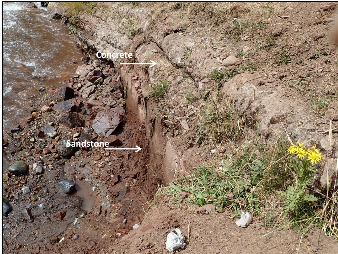
Photograph 7: Sandstone and concrete bank reinforcement, looking south-west
