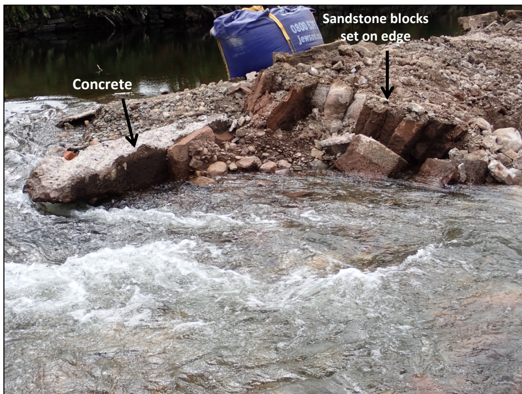
Photograph 6: Detail of section through the weir, looking south-east
