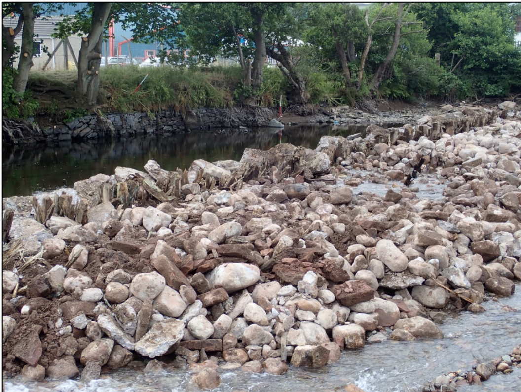
Photograph 14: Cobbles forming the surface of the weir (disturbed by the removal of the modern concrete), looking south-east
