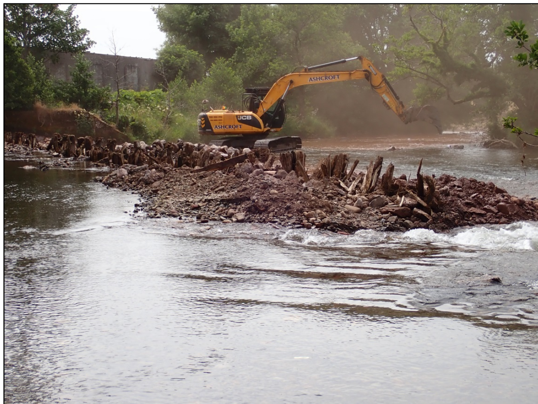
Photograph 10: Upright timbers and planks forming the front (east side) of the weir, looking south-west
