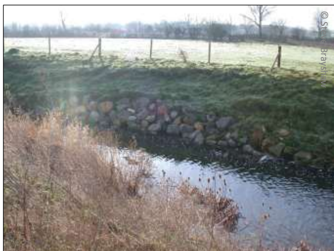
Fig 7. Large rock bank toe protection
