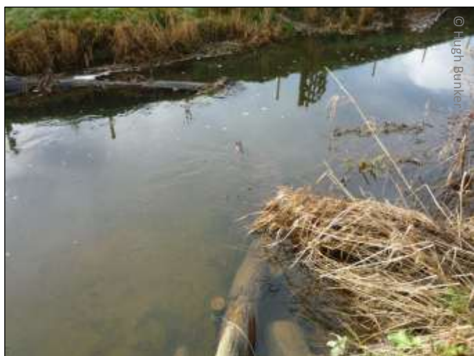
Fig 3. Woody debris deflector
