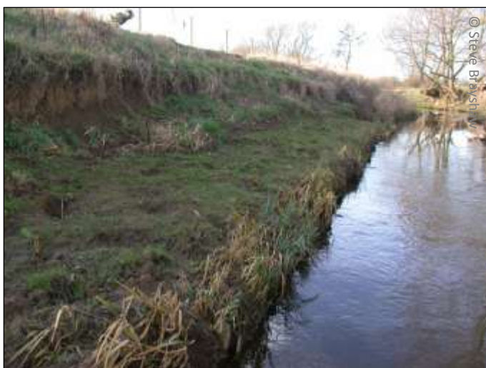
Fig 8. Pre-planted coir bank toe protection backfilled with earth
