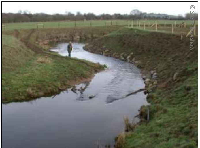
Fig 16. The meander before and after, showing new paired faggot deflectors, bank stabilisation and fencing
