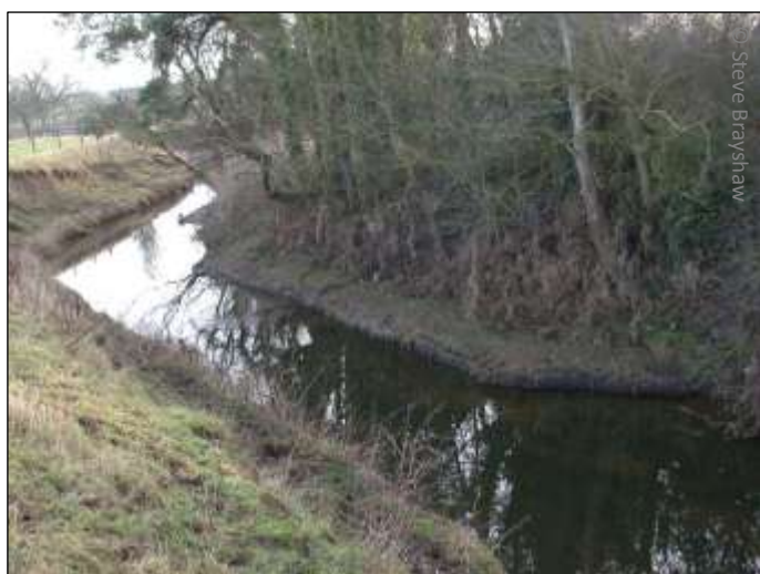
Fig 5. Earth-filled faggot and coir pinching
