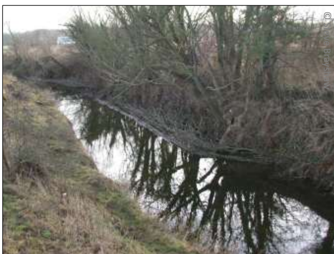
Fig 6. Faggot pinching back-filled with brash to trap silt
