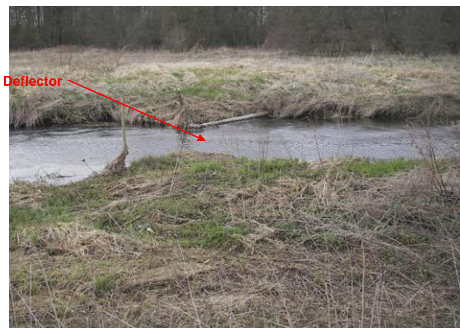
Plate 2 - A deflector installed in Reach 19. This deflector was not substantial enough to be effective (source: RRC, 2007)
