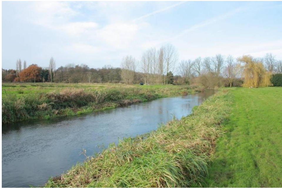
Plate 13 - A section of river in Reach 18 which has been straightened, widened and deepened
