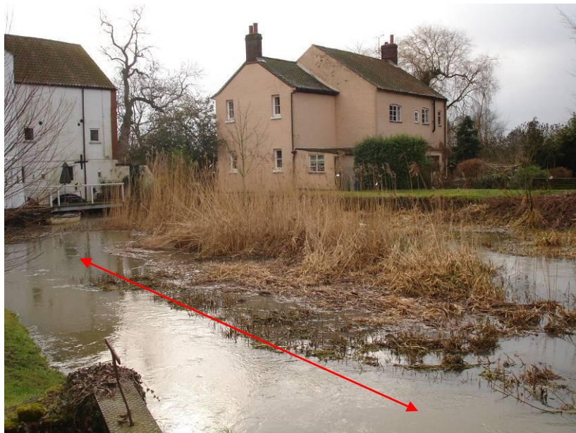
Plate 11 - Accumulated silt in main channel (as depicted by the arrow) immediately upstream of North Elmham Mill, Feb 2009
