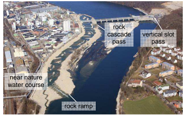
Figure 19. River Rhine, Rheinfelden (D): New power plant designed as run-of-river type. Near-nature water course installed in the old headrace channel.
