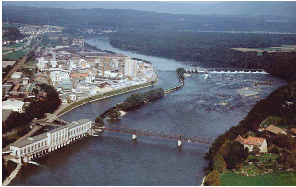
Figure 18. River Rhine, Rheinfelden (D): Old hydrolic power plant designed as diversion type.
