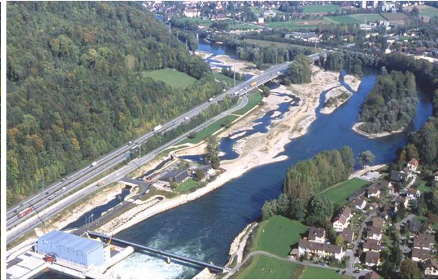
Figure 8. River Aare, Ruppoldingen (CH): New hydroelectric power-station. The headrace channel was filled up and a nature-like river was installed.
