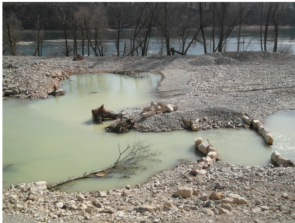
Figure 22. River Rhine, Rheinfelden (D): Typical elements: riffle made of gravel and stone, deeper flow path (blocks) and structures of deadwood.
